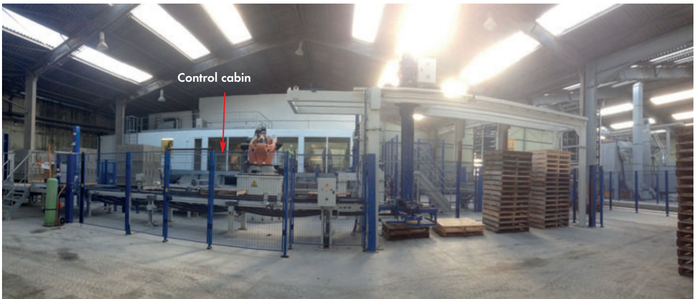
At the heart of the facility is a noise-insulated control cabin located in the middle of the production line.
