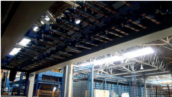
Automatic steel reinforcement insertion.
