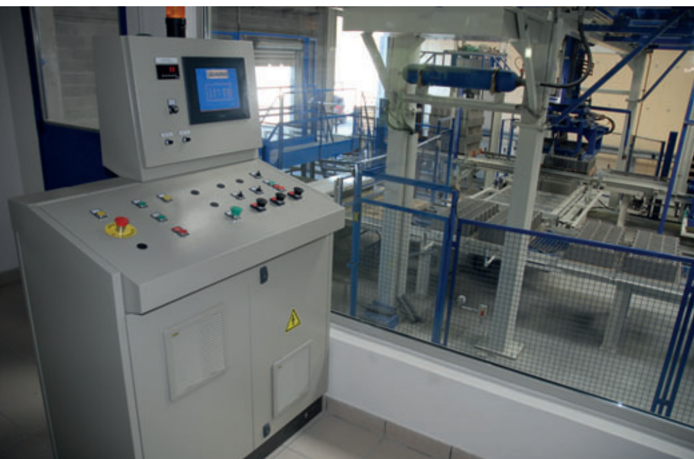
Insulated control cab with large windows which allow a perfect view of the plant
