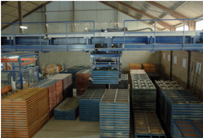
The overhead travelling crane is equipped with an on board PLC
