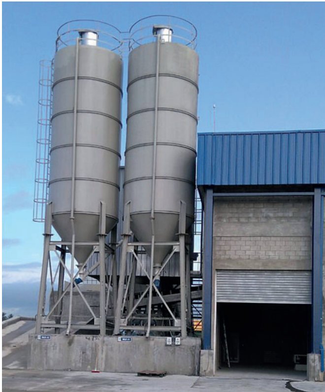
The batching plant is fully galvanized and is built above the ground level
