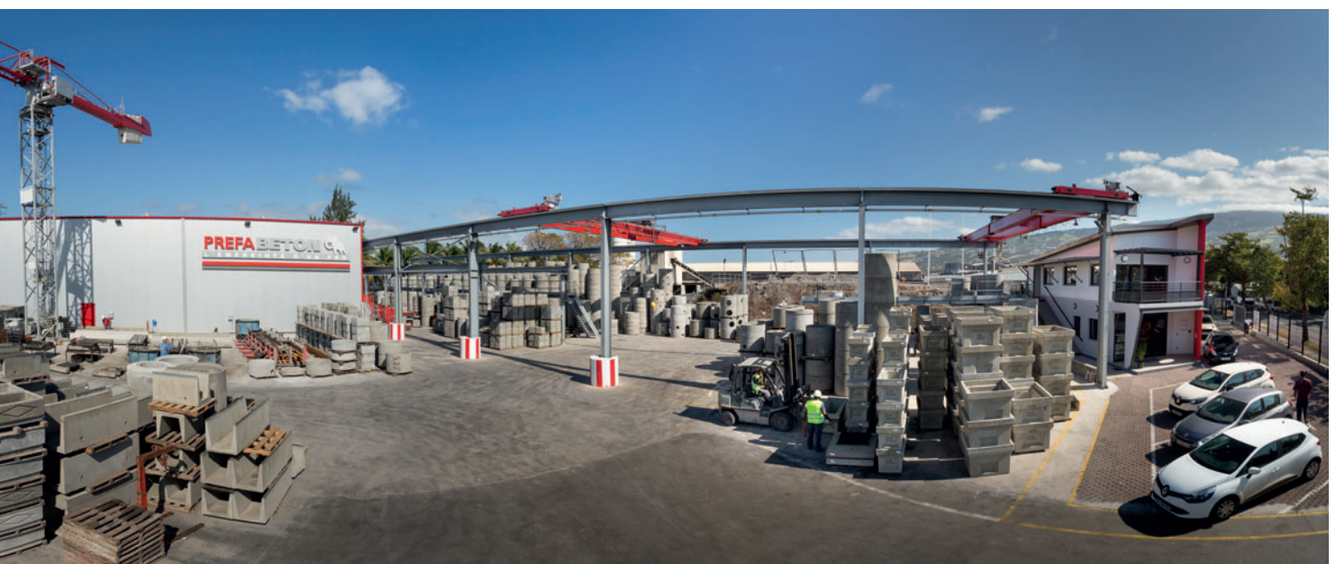
Fig. 1: Prefabeton, one of the leading manufacturers of concrete product on the Island of Reunion
