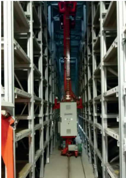
Fig. 7: Automatic storage and retrieval machine
