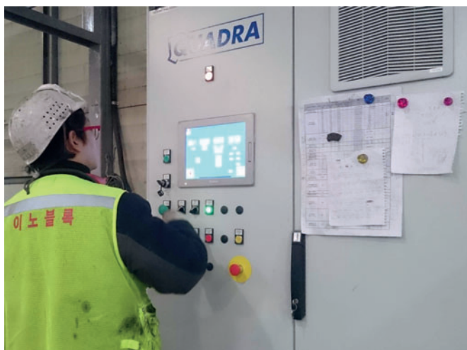
The PLC program designed by Quadra allows the backup and the automatic recall of the dosing settings
