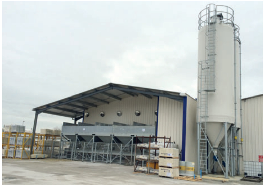
Batching & mixing plant
