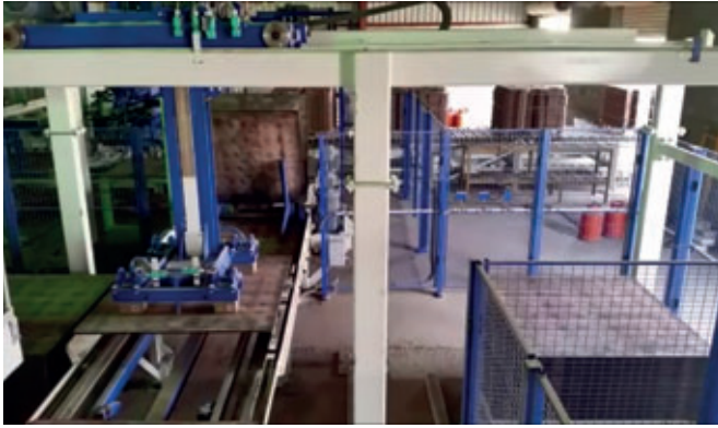
Pallet buffer with 600 pallets stored.
