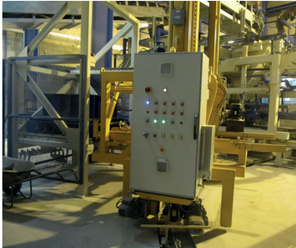
Depositing the mould close to the block machine
